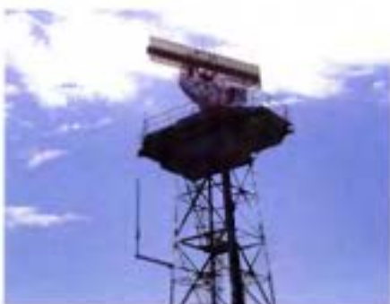
Figure 2 (above). Different ADS-B track symbols are used to convey the level of accuracy and reliability of data. Figure 3 (top right) compares red ADS-B tracks and green radar tracks for four flights. In Figure 4 (right) the ADS-B antenna can be seen mounted on one side of the Brisbane Airport radar tower.
