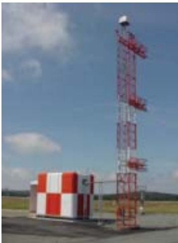
Flight inspection of an ILS installation involves checking the accuracy of signals transmitted by a localizer antenna (Figure 1, above), and a glide slope antenna (Figure 2).
