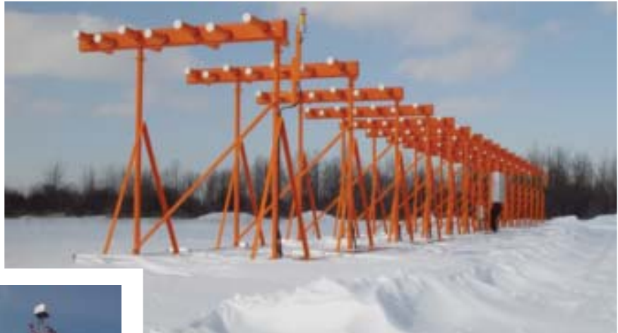
Flight inspection of an ILS installation involves checking the accuracy of signals transmitted by a localizer antenna (Figure 1, above), and a glide slope antenna (Figure 2).
