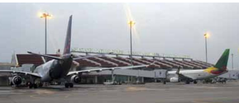
Tarmac Yaoundé-Nsimalen Airport
