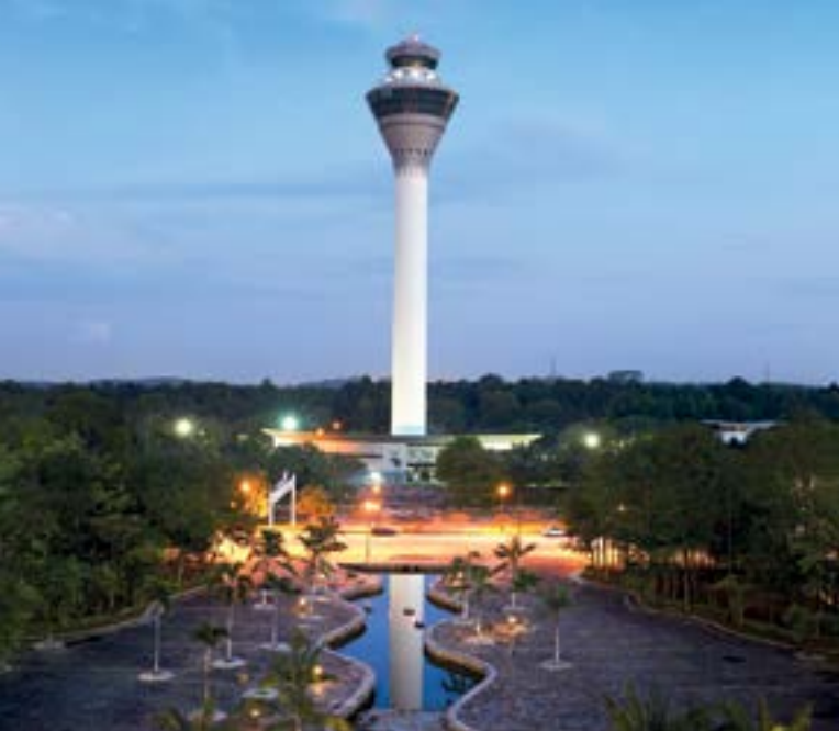
DCA Tower at Kuala Lumpur International Airport
