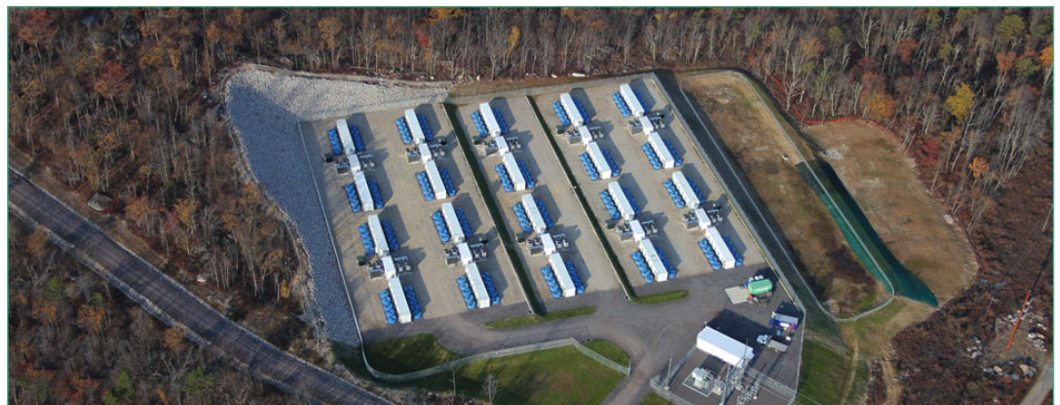
FIGURE 2-19 A facility in Pennsylvania comprised of multiple flywheels to store electricity (source: Beacon Power)
