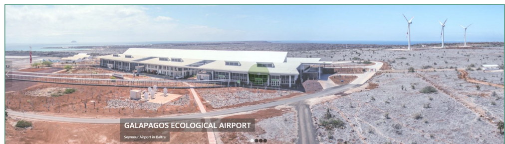
FIGURE 6-1 Seymour airport's wind turbines and solar panels atop walkway canopies (source: Ecogal S.A)
