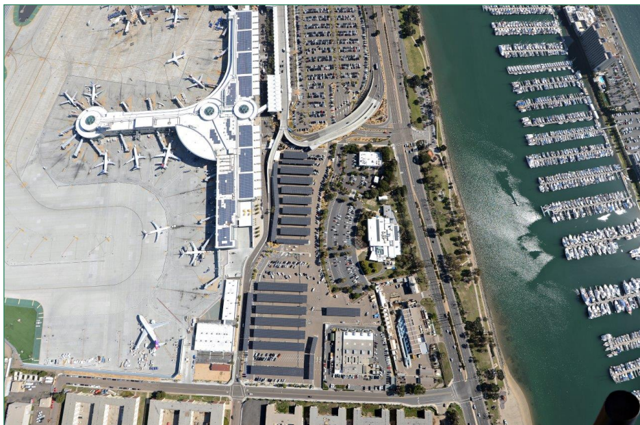
FIGURE 6-7 Solar project at San Diego international airport (source: San Diego County Airport Authority)
