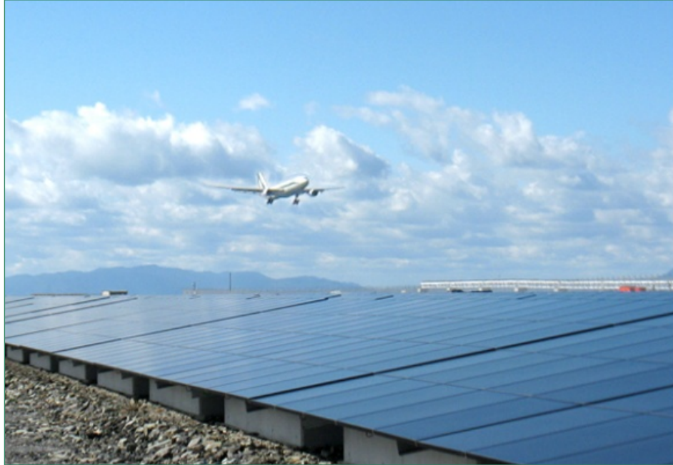
FIGURE 6-8 Kansai international airport solar facility on cargo warehouse (source: Solar Frontier)
