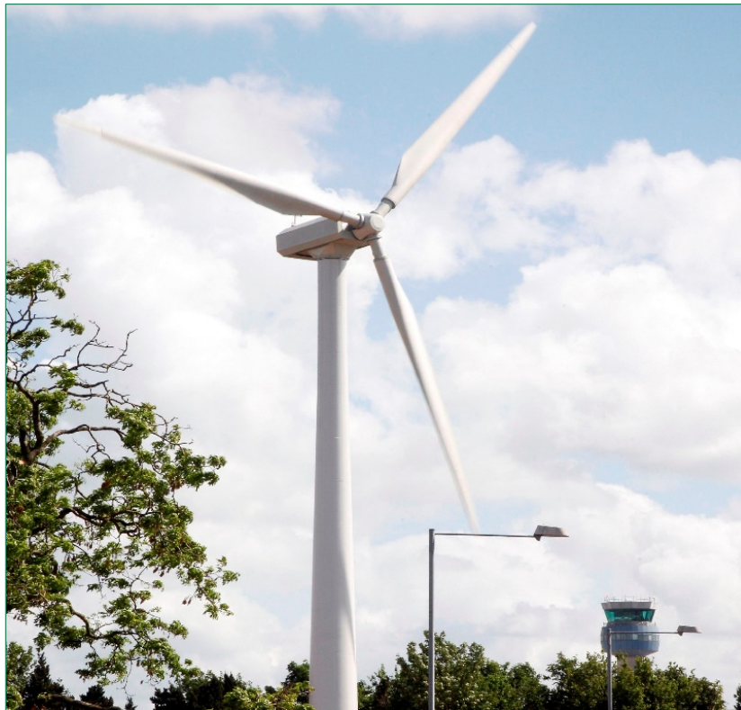
FIGURE 6-2 One of two wind turbine generators at East Midlands airport (source: Manchester Airports Group)
