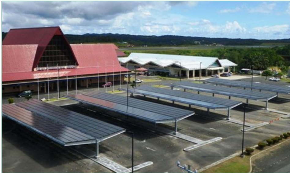
FIGURE 6-6 Palau international airport solar facility (source: Solar Feeds)
