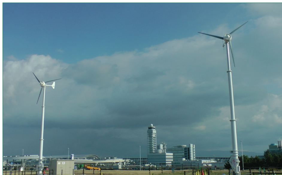
FIGURE 6-9 Wind turbines at Kansai international airport (source: Zephyr Corporation)
