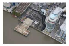
**Figure 3:** The London Heliport at Battersea. The landing surface is located on a platform just off the banks of the Thames River and, depending on the tide, is classified as either a surface-level or elevated heliport. Making an approach even more challenging, the London Heliport is closely surrounded on the banks of the Thames by mid-rise buildings.
