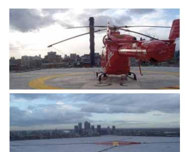
**Figure 4:** The Heliport at London's Whitechapel Hospital. While the photo showing the proximity of a smokestack to the existing helideck (*top*) provides a quintessential example of the kinds of obstacles that make operations in urban environments dangerous, the new helideck under construction (*lower image above*) rises well above most of the nearby city skyline at 17 storeys above street level, providing a perfect perch to capture a beautiful evening view of London.
