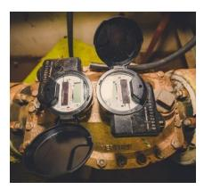
Water metering is necessary for managing water use more effectively by detecting leaks and improving the accuracy of unaccounted and unmetered usage. In 2017, the Airport Authority installed new water meters in all terminal buildings (Figure 2). The Airport Authority has also improved water metering of its irrigation system.
